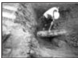
Inspection of pipeline puncture and close-up of damaged area.
